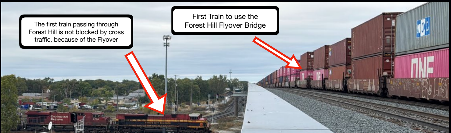
The first train crosses the new bridge without impeding traffic below.
