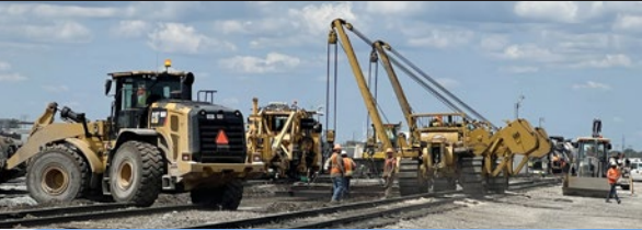
Machines are used to place a track panel.
