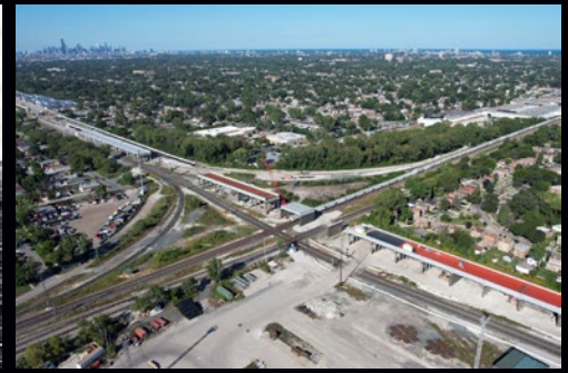
The Forest Hill Flyover project in progress.
